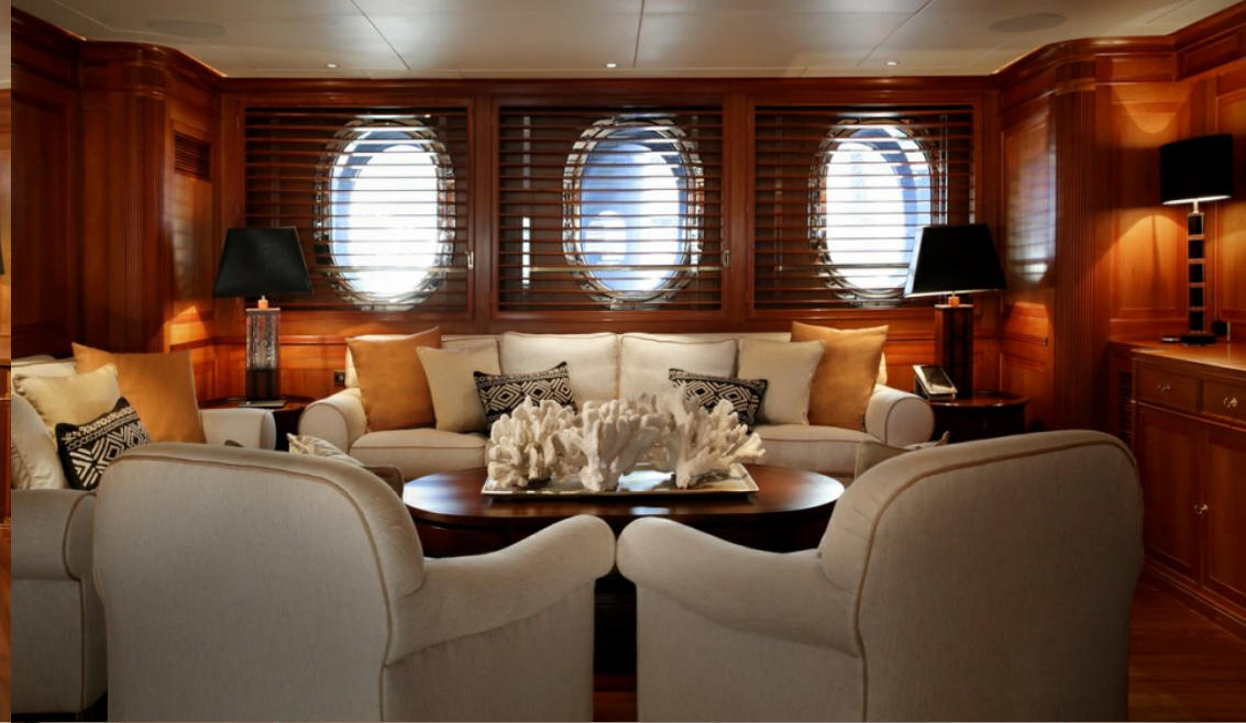
Lower deck lounge
